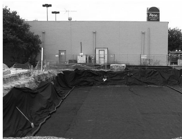
Place non-woven geotextile over prepared soils and up excavation walls.
