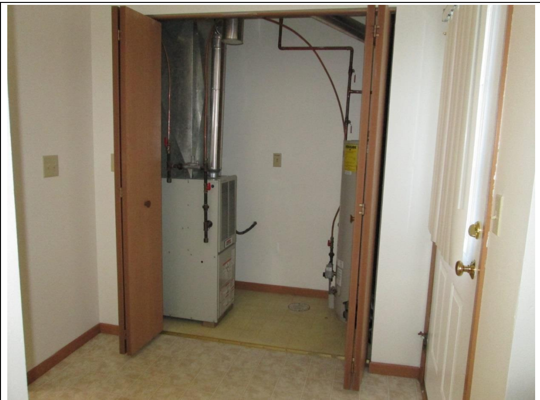
Photograph #15 West Birch Estates & Proposed 16-Unit Apartment B1800529.00 Date: February 1, 2018 BRAUN INTERTEC Location: Inside a vacant unit Subject: Typical natural gas forced air furnace
